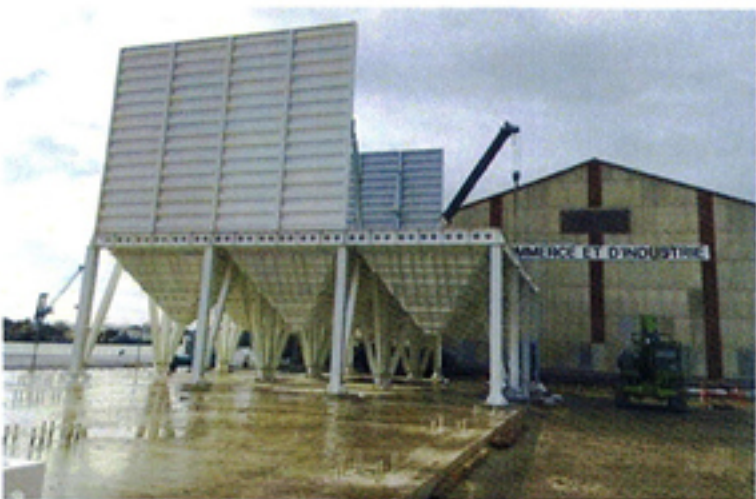
Installation of cement silos.
