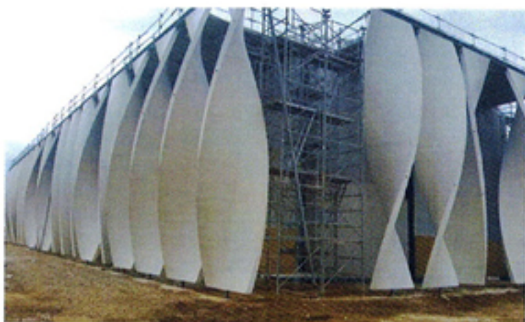
Precast concrete facade of multi-sports hall building for a polytechnique school in France.
