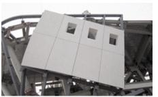
The GRC panels from the roof system to each of the layers of floors were designed in a unified diagonal line, which increased the difficulty of its installation, considering the partition of the glass windows and connections. Thanks to the latest technologies of BIM (Building Information Modeling) to monitor the process from design and production, this high-precision GRC project became successfully completed in late 2016.
